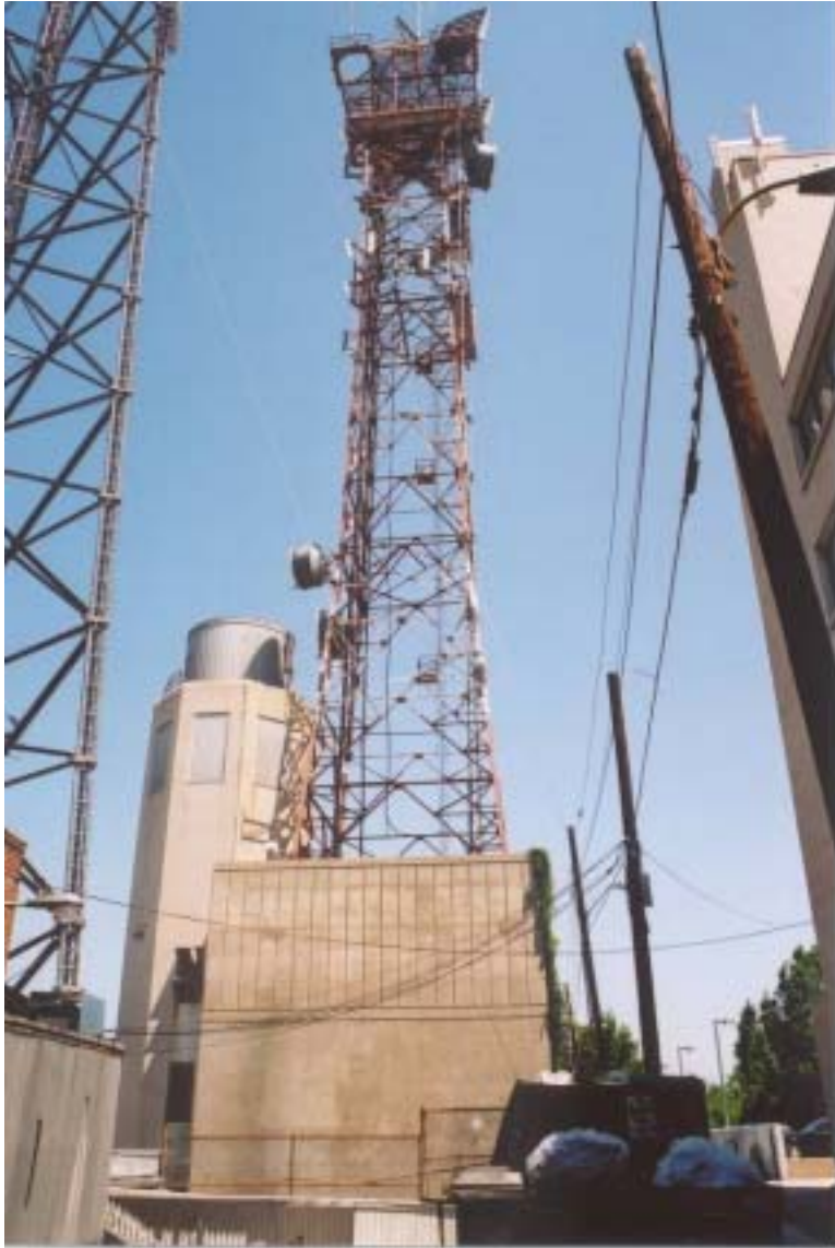
Western Union Telegraph Company Tenley Tower: 1963 third-story addition and tower. View to the north.
