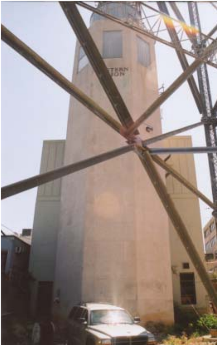
Western Union Telegraph Company Tenley Tower: West Façade.
